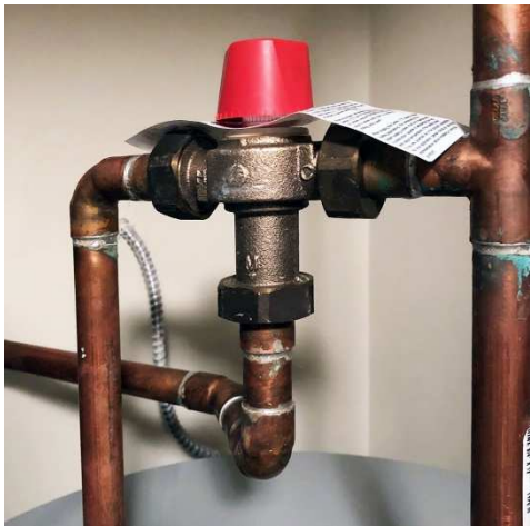
The mixing valve is below the red cap
